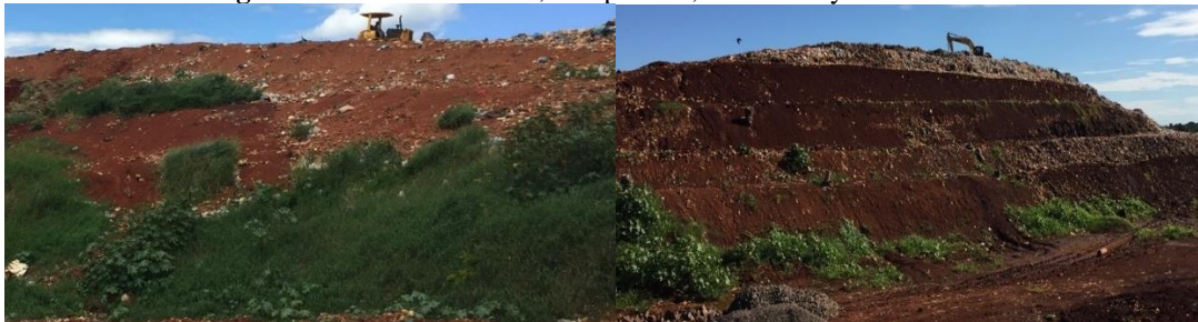
Figure 8 - Accommodation, compaction, and overlay of the waste.
