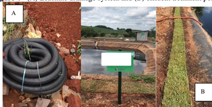
Figure 4 - (A) Leachate drainage system and (B) effluent treatment ponds.
