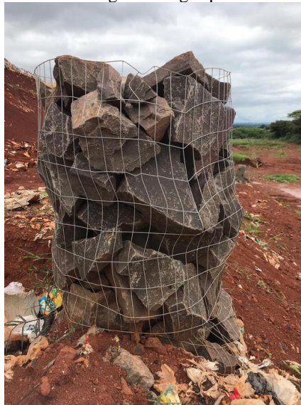
Figure 6 - Drainage of the gas present inside the landfill.
